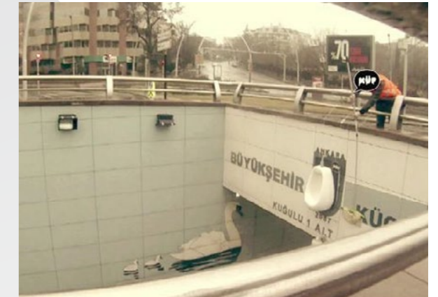
10. Urinal Installation by KÜF Project, 2011
